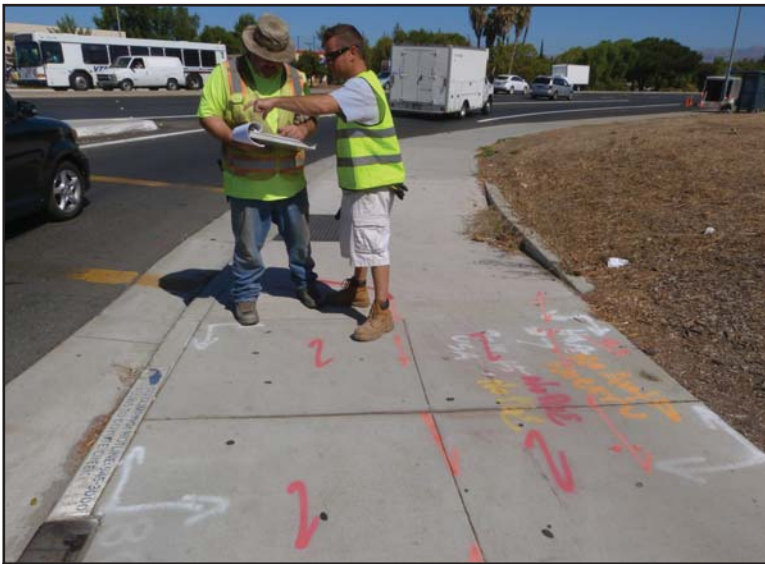
Photo 1. Core 7, an example of a location that was previously heavily disturbed by electrical lines and a nearby drain system, and so could not be safely cored.
