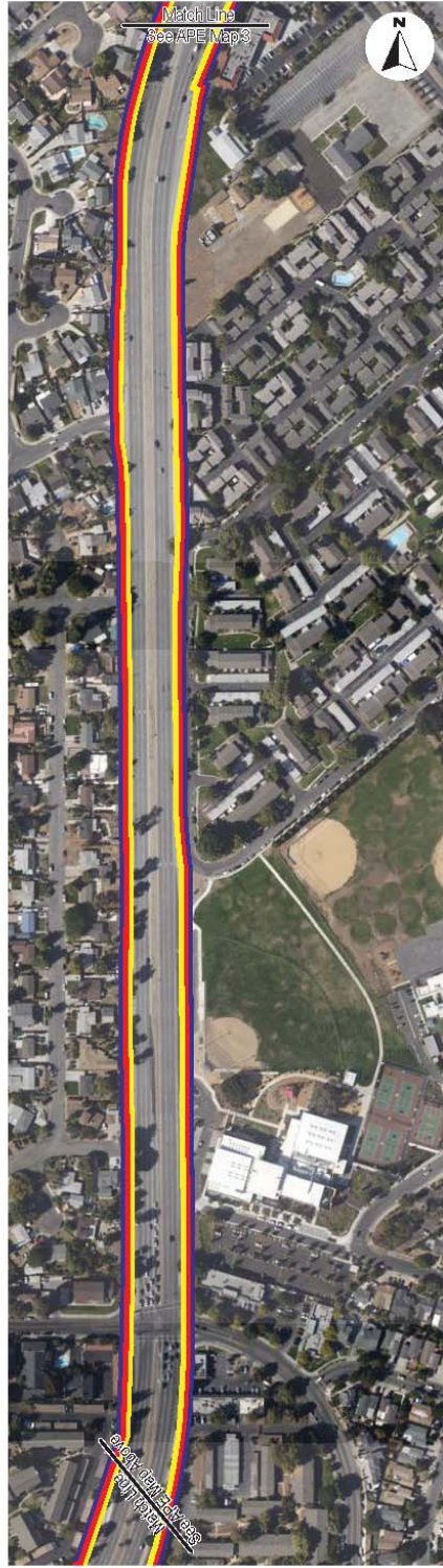
Capitol Expressway ITS & Sidewalk Project, San Jose, Santa Clara County: CML 5937 (196)
