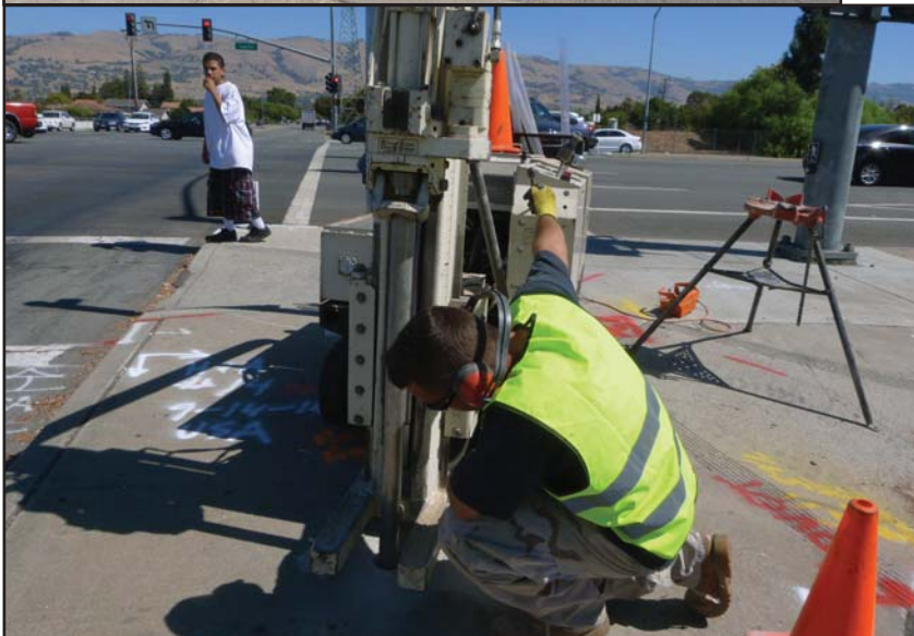
Photo 3. In progress photo of sampling at Core 14.
