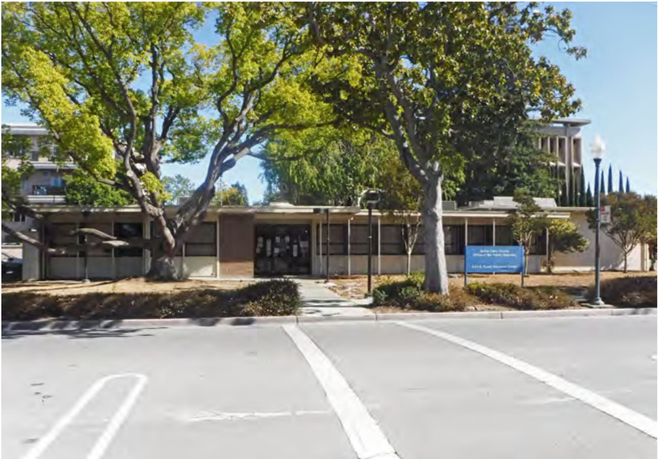
Photograph 1. Office Building at 231 Grant Avenue, view to southeast from Grant Avenue
