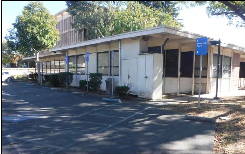
Photograph 4: North end of façade and northeast side, camera facing south, September 23, 2020.
