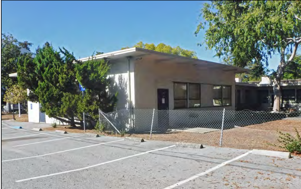
Photograph 10: Southwest and southeast sides of building, camera facing north, September 23, 2020.
