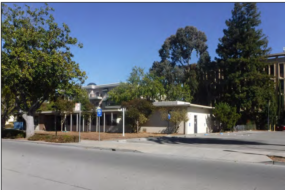
Photograph 11: Façade and southeast sides of building, camera facing east, September 23, 2020.
