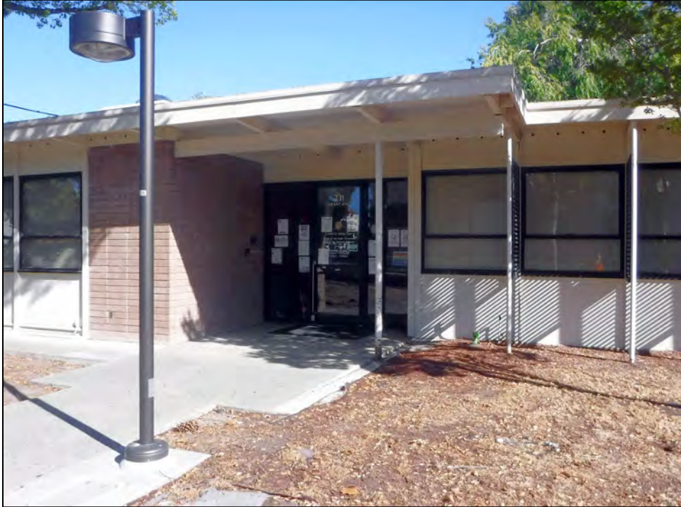
Photograph 2: Detail of primary entry, camera facing east, September 23, 2020.
