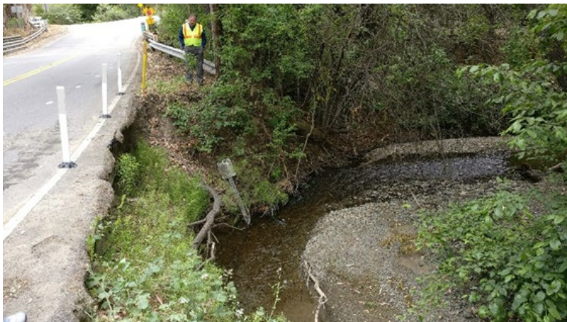
FIGURE 1. ARASTRADERO ROAD BEFORE OCTOBER 2017 EMERGENCY REPAIR
