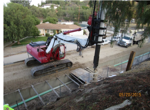
FIGURE 3. DRILL RIG INSTALLING SOLDIER PILE WALL FOOTINGS
