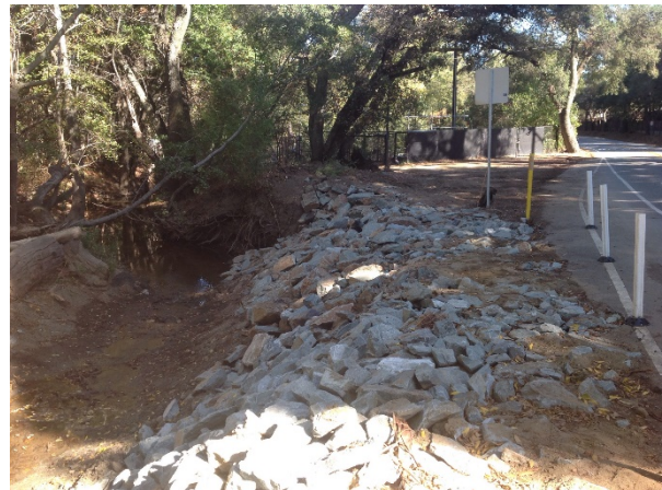
FIGURE 10. RIPRAP INSTALLED ADJACENT TO ARASTRADERO ROAD DURING EMERGENCY REPAIR
