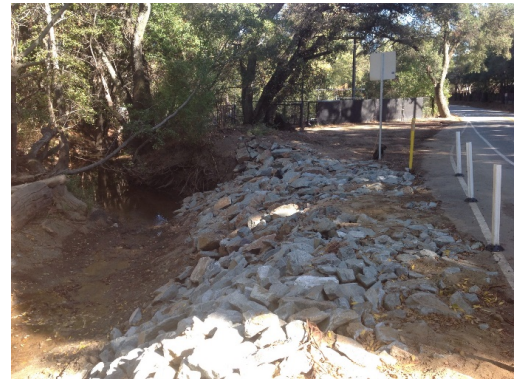
FIGURE 2. RIPRAP INSTALLED ADJACENT TO ARASTRADERO ROAD DURING EMERGENCY REPAIR
