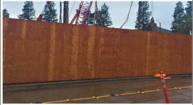
Top: 10-foot-tall barrier consisting of double  $\frac{3}{4}$ " plywood affixed to 6 x 6 posts driven into the ground. Bottom: Solid exterior face of the same 10-foot-tall barrier. Image Source: MIG.
