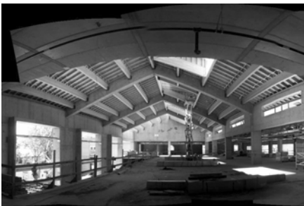
Below: Construction of the new Gilroy Library
