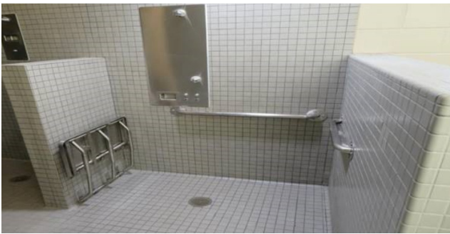
(This image is highlighting inmate restroom improvements for inmates requiring Americans with Disabilities Act (ADA) mobility needs.)
