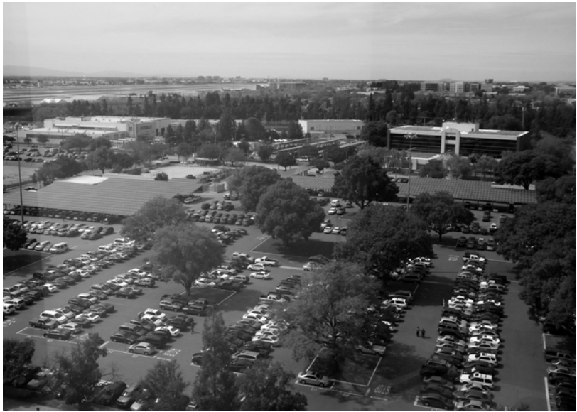
County Government Center-Solar Panels
