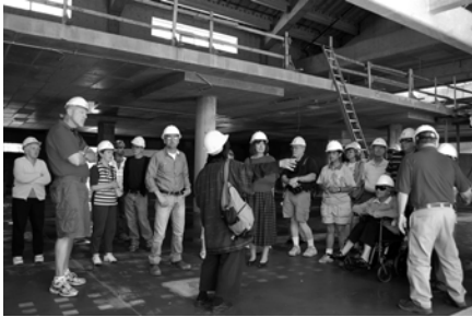
Below: Construction of the new Gilroy Library
