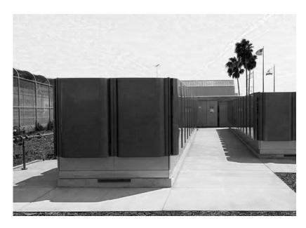
The Fuel Cell system installed at the Elmwood Correctional Facility is an 800 kilowatt system that generates 7 million kilowatt-hours of clean electricity each year, while saving the County an estimated \$2.5 million over the 20 year Power Purchase Agreement under which it was installed.
