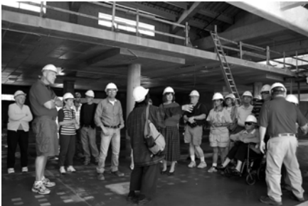
Below: Construction of the new Gilroy Library
