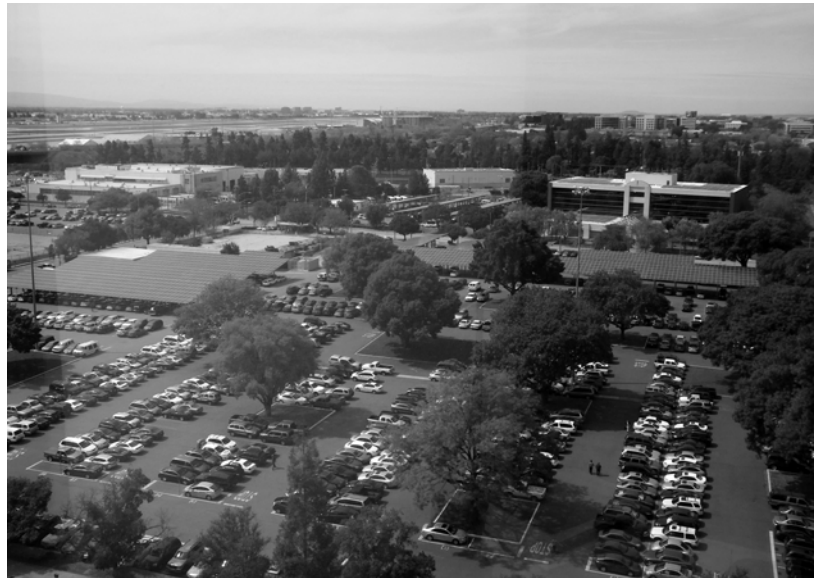
County Government Center-Solar Panels
