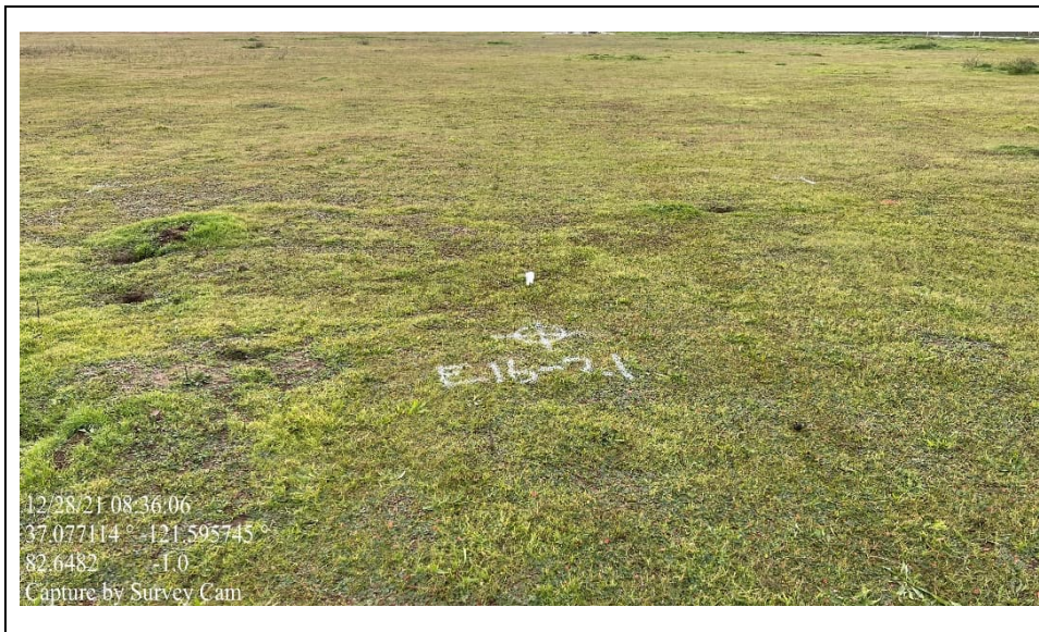
12/28/2021. E16-21: Utility Clearance
