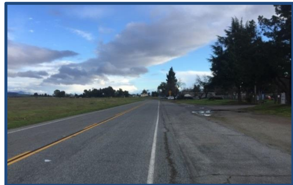
Murphy Avenue looking south
