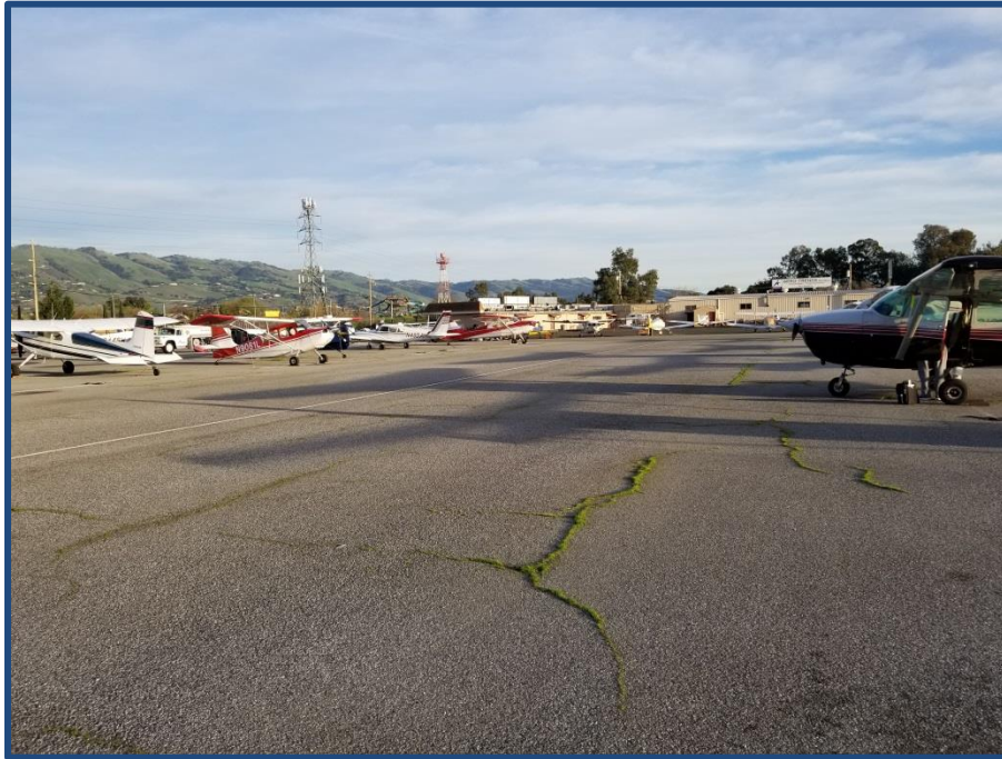
South taxiway looking east.
