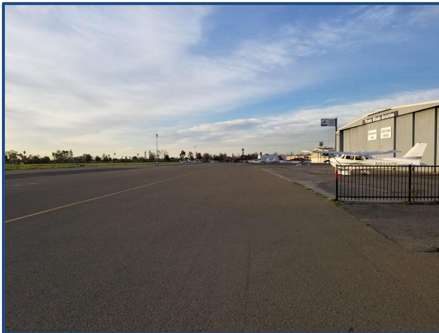
Southwest area of subject, looking north.
