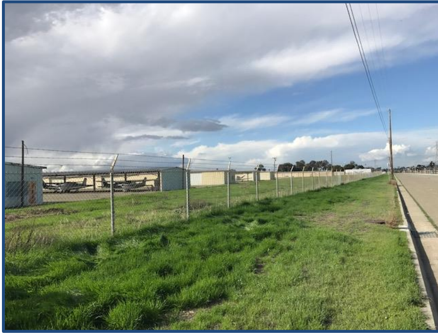
View of Subject Property from Swift Avenue
