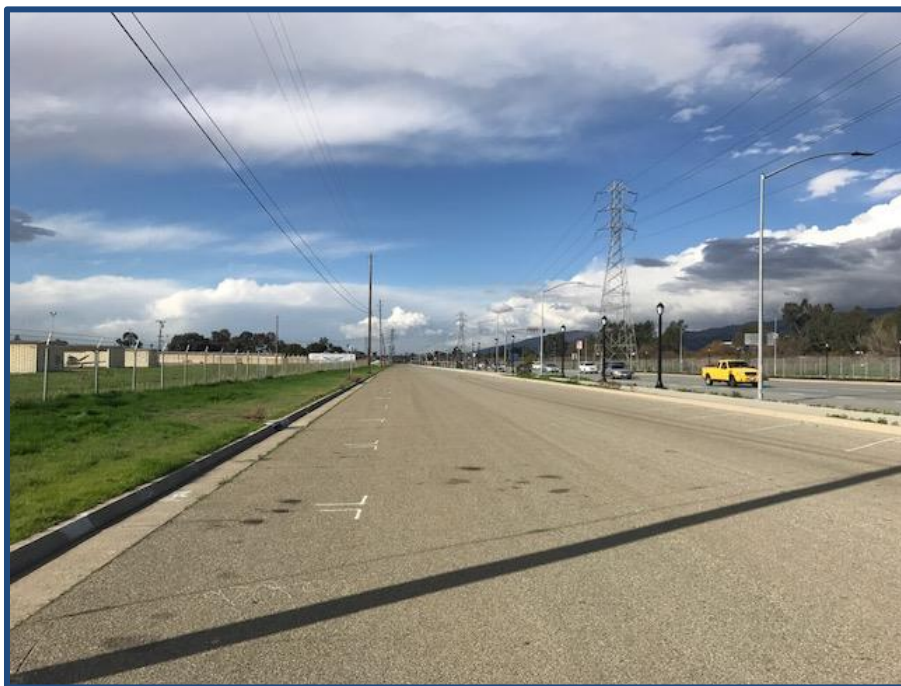
View of Swift Avenue frontage
