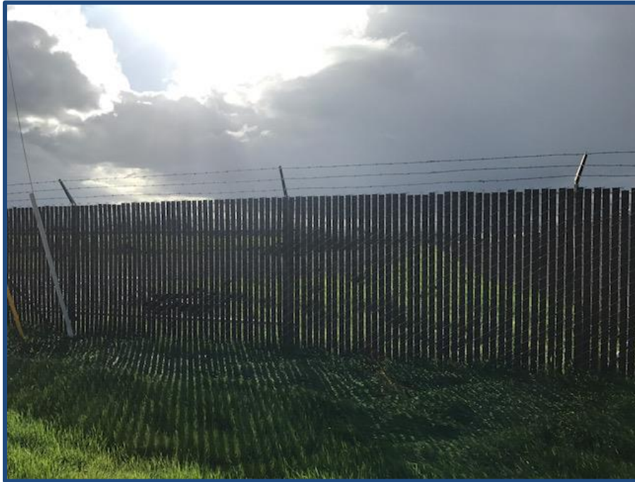
View of the fence which perimeters the subject along Swift Avenue and Swift Lane
