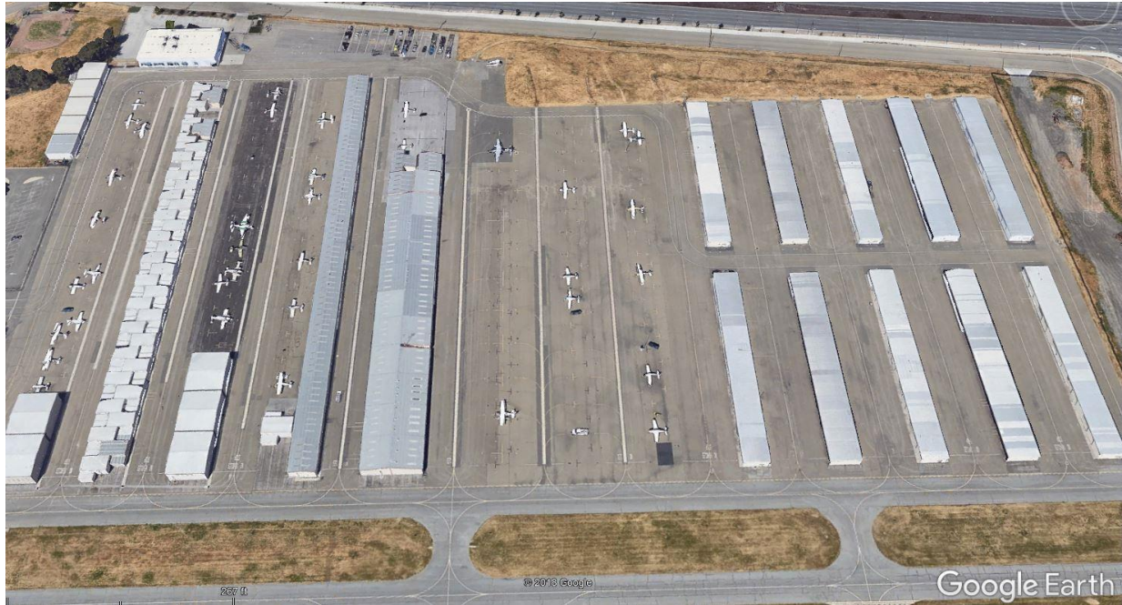
Figure 2 – There are only 37 planes tied down on the county ramp, along with nearly full shelters and hangars. Tie downs provide much less revenue than shelters and hangars. It is good to have vacant ramp space which can be used in an emergency for extra helicopters, planes, commodity points of distribution and/or tent cities for emergency workers. Lost tie down revenue is recovered through marking leaseholders rates to aviation market. It is fine to leave the majority of planes on the northeast side.
